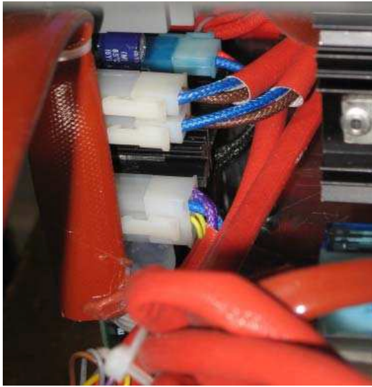
Thermal protection of power transformer
