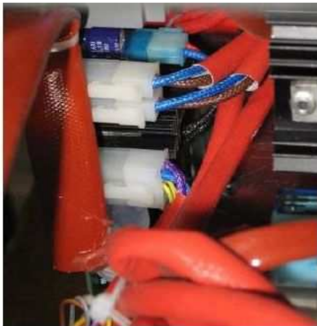
Thermal protection of power transformer
